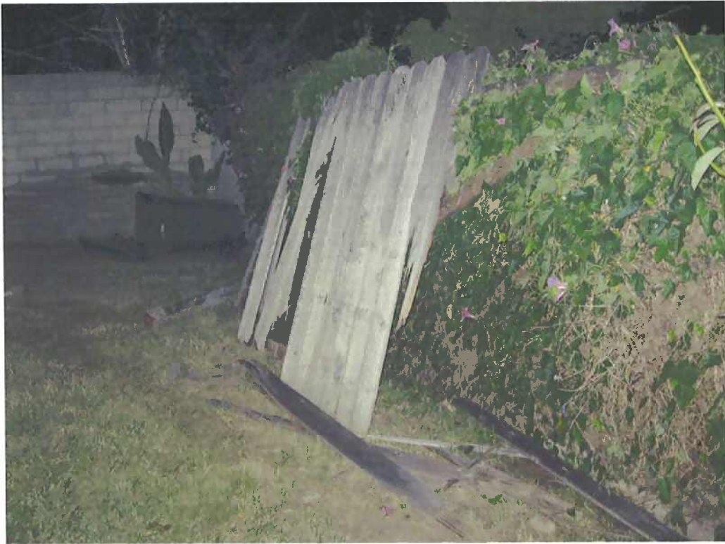
Gate in backyard
